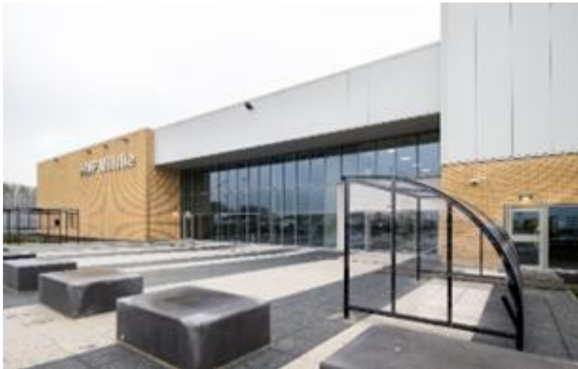
HMP Millsike - Entrance Building 1
